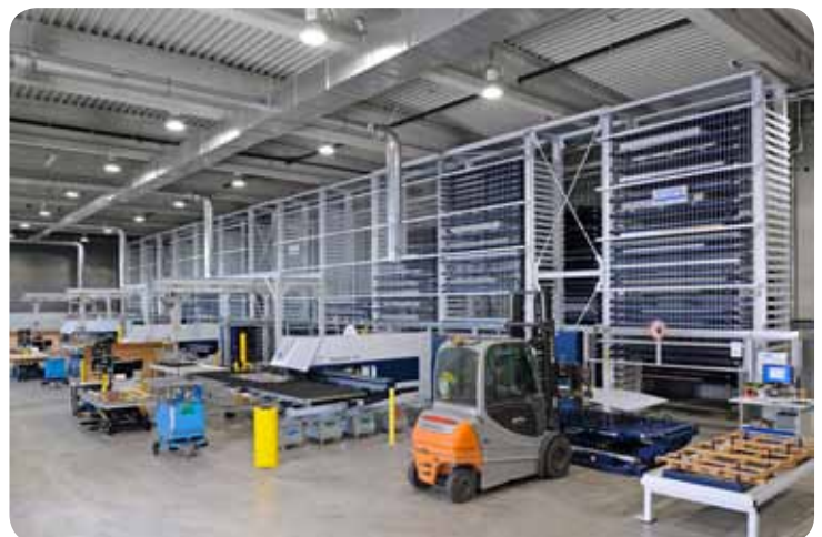
The forklift truck places the sheet stack on the deposition plungers of the incoming goods station. The sheet stack can thus be positioned without being damaged and the fork attachment withdrawn again very easily.
